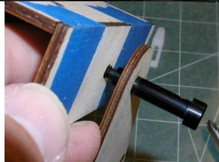
Add the nut to the inside and tighten securely.
